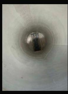
sulfide (H2S). Debris would get stuck on the exposed metal creating an increase in the H2S and the two manholes were at the high points on the sewer and the gas would get trapped in the chimney section.
