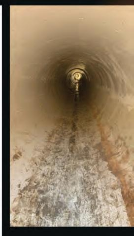
Wallingsford, based on his many years in the sewer and water sector, was aware of cured-in-place pipe (CIPP) and other trenchless rehab methods, but none he knew of would work on a pipe as deteriorated as this. "In my experience, CIPP would blowout when it got to the collapsed section of pipe, but he [the contractor] was persistent on getting the company [with the new technology] out to look at the pipe," Wallingsford said.
