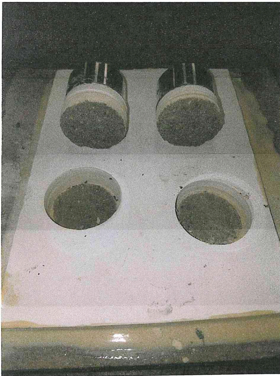
Figure 6: 50mm test dollies pulled using Elcometer 506 adhesion test unit, and visible substrate failure.
